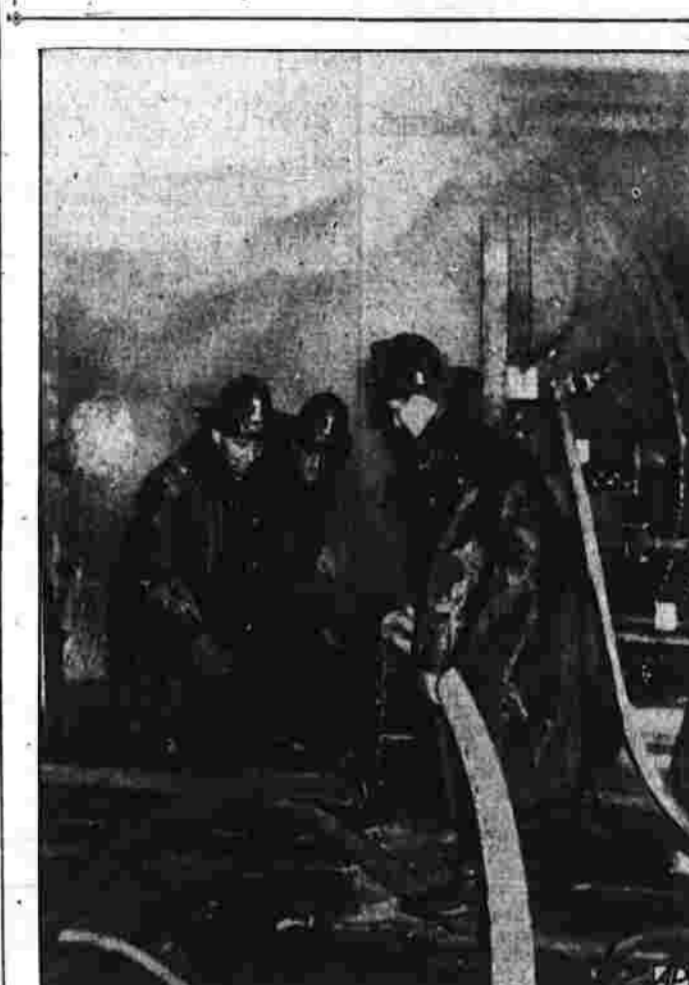
After a stubborn battle, New York city firemen succeeded in quenching a blaze in the north bore of the Manhattan-Queens 455-1000-foot vehicular tunnel under the East river. The fire broke out in construction timbers near the air-lock where "sandhog" work under pressure of 48 pounds to the square inch, 150 feet below the surface.
